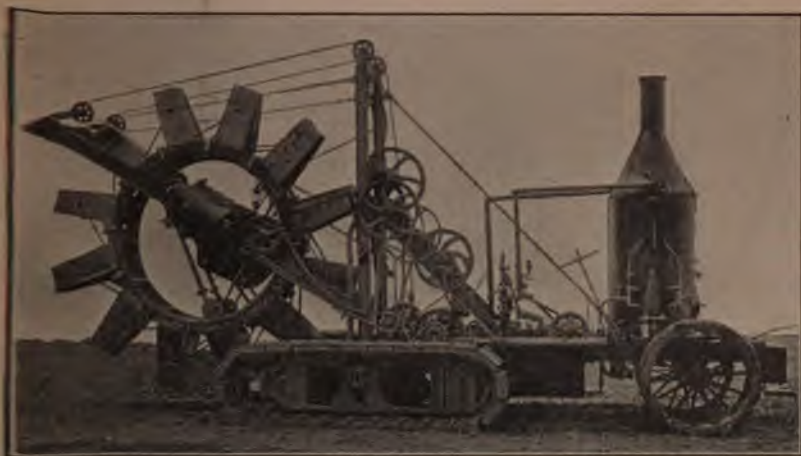
Wheel Excavator. Figure 63.
